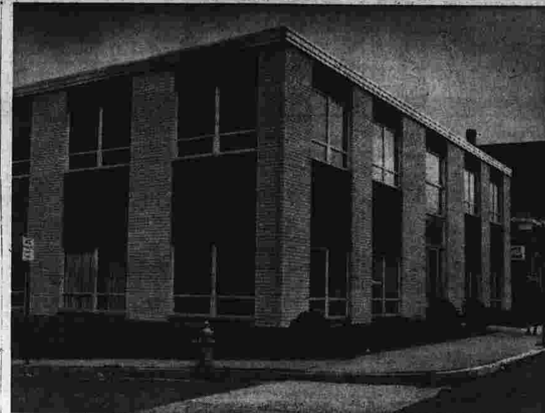
The Willard Building, Manchester's newest office building at 320 Main St., is of red and yellow brick construction with frame floors. John R. Wennegren Co., general contractor, is completing the exterior of the building as desired by the occupants, of which there are now five, the latest being the main offices of Mark Kravitz and Bernard Hickey, doing business as "Hob-Nob, Inc." a restaurant chain in New England and Puerto Rico. The two-floor structure, which has better than 9,000 square feet of office space, was designed by Arnold Lawrence, architect. Weyerhaeuser "Craft-Wall" paneling, a new product in this area is being used in exterior walling. A feature of the building is the gas heating and air-conditioning elements, installed on the roof to provide more inside office space. Simulated glass is also being used. The G. H. Willard Co., owner of the office building, reported a parking area to accommodate 30 to 35 cars will also be available. (Herald photo by Finke).
